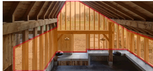
Fig. 03. Interior of The Sixteen Oak Barn: Natural Ventilation
